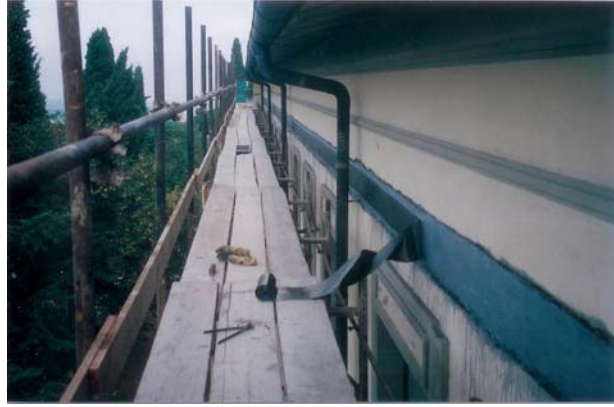
Strengthening using carbon fiber sheets of the structural walls
