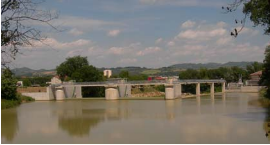
Overall view of the dam
