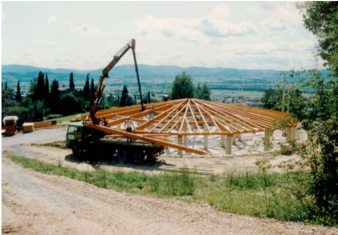
Installation of the glulam roof structure
