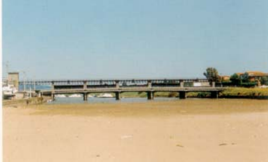
5 span bridge view
