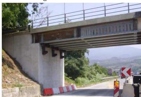
Strengtheneng view of the bridge before final painting of the beans
