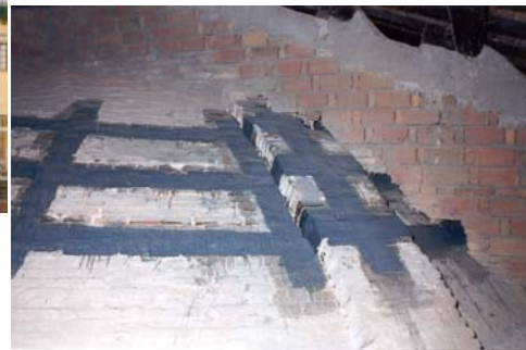
View of carbon CFRP fiber installation
