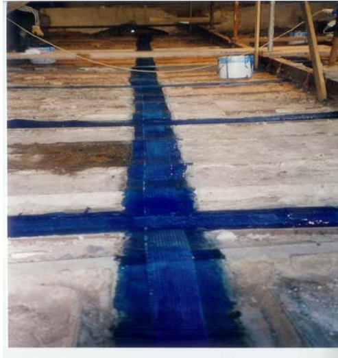
Retrofit job of the vaults using carbon fiber sheets
