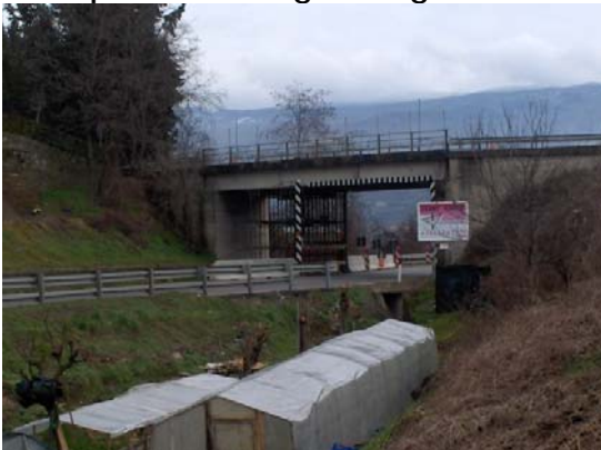
view of the bridge
